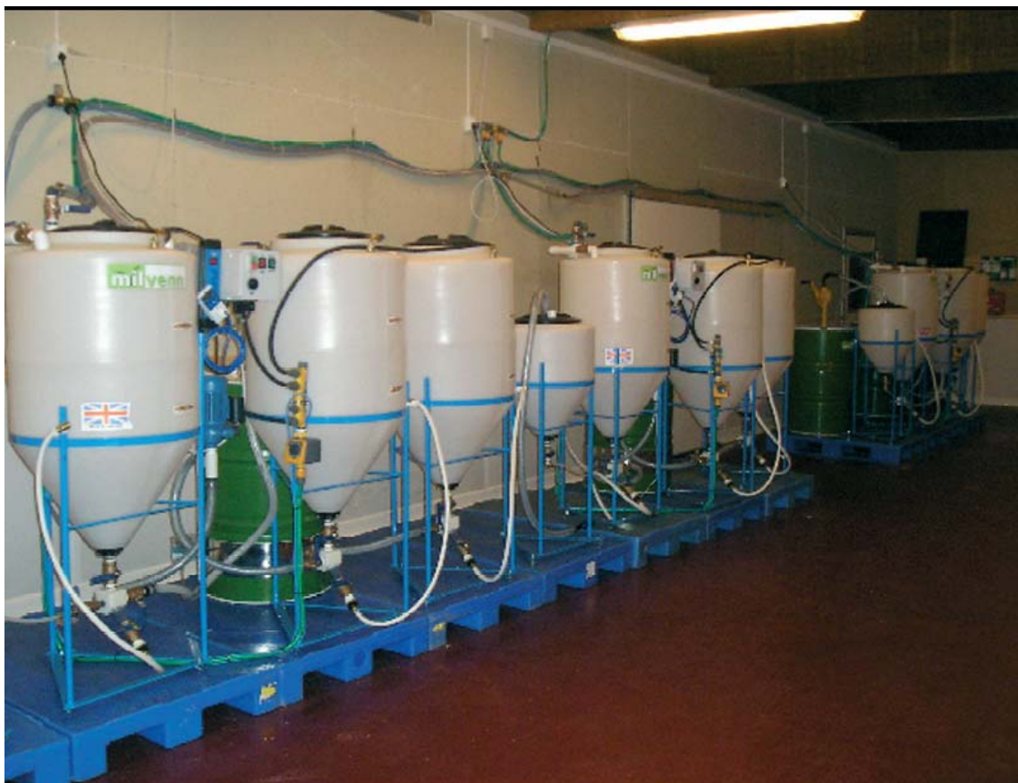
Figure 3 From the Milvenn production facilities
