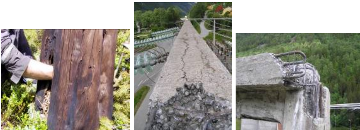
Images 4-6 Examples of ageing in technical components, a high-voltage power mast on the left and two low-voltage power masts on the right. The age of these two types of masts generally being the same, the DCPEP assume that high-voltage masts are in an equally poor condition as the depicted low-voltage masts. These particular masts have now undergone repairs. 137
