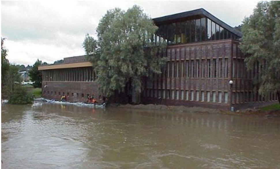
Figure 14. The rescue service is making temporary embankments to prevent damage to the public sports hall during the flood in 2001. Source: Sundsvall Municipality
