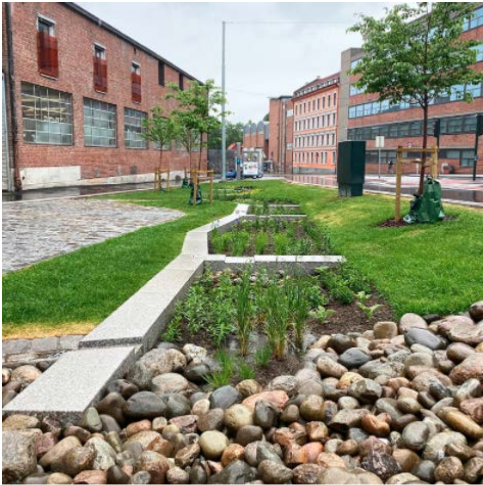
Figure 18. Rain garden established on earlier sealed surface. Photo: Tharan Fergus, Oslo Municipality
